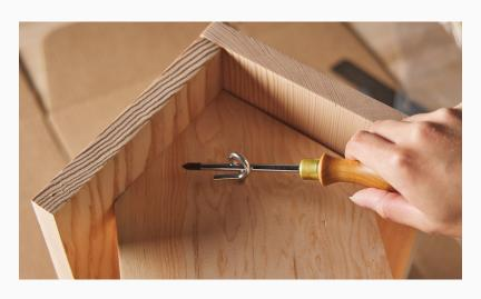
d. Loop each end of the chain into a loop hook.
